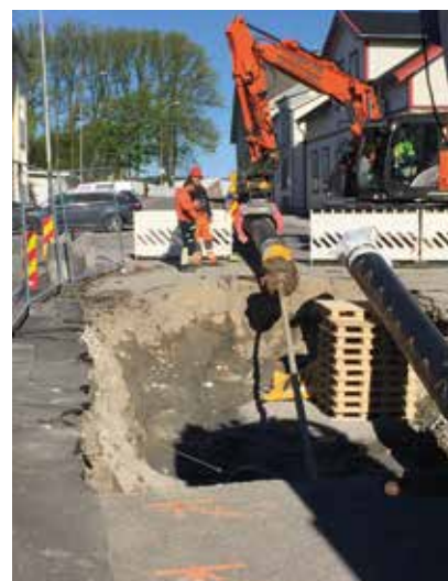
Borestreng for styrt boring.
